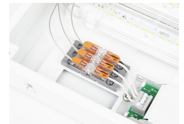
Multi-pole, fixed lighting fixture wiring
